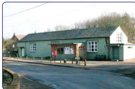
Helions Bumpstead Village Hall before
