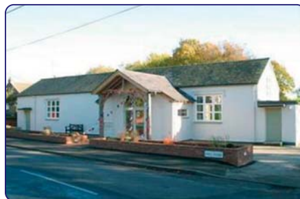
Helions Bumpstead Village Hall after
